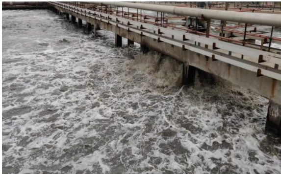
Figure 6: Aeration Tank
